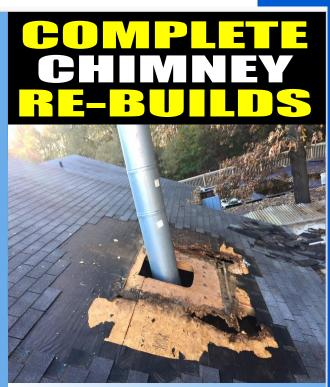
Complete tear down and re-build of the chimney frame around the flue pipe. Install new OSB walls and a underlayment. Install new chimney flashing and cover flashing with underlayment, then wrap chimney with a moisture wrap and install
