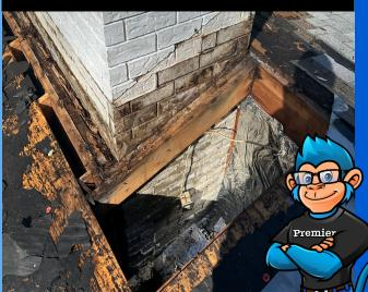
We Completely tear off the shingles and any old flashing around the chimney. Then we inspect and replace any bad wood found on the roof system. Next we install new roofing underlayment and new custom made chimney flashing and seal. Next we install new shingles to match your existing roof system and clean the work area. Last we remove the project trash and remove from property.
